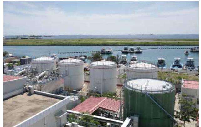
Figure 8 - Hulhumale' Fuel Storage Tanks
