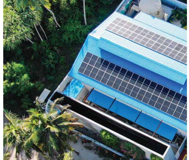
Figure 1 - Solar Installation STELCO Powerhouse rooftops
