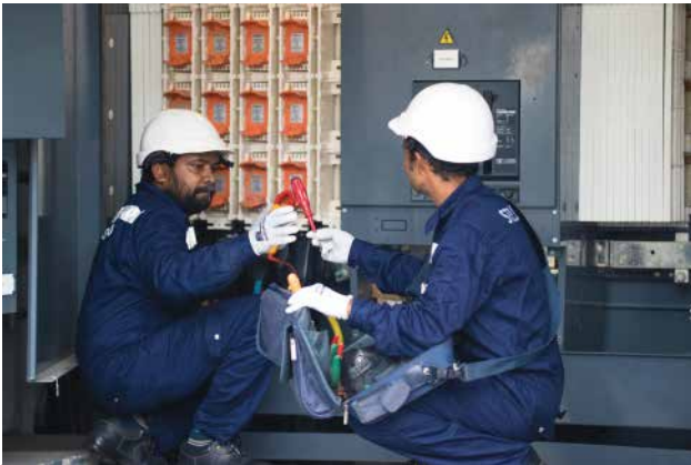
Figure 16 - Substation Maintenance works
