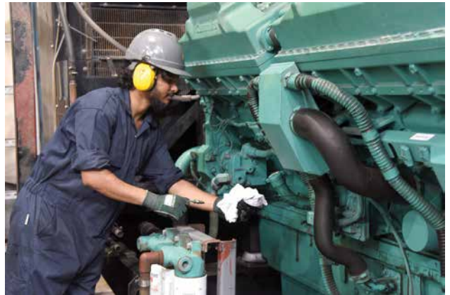
Figure 17 - Generator maintenance works ongoing
