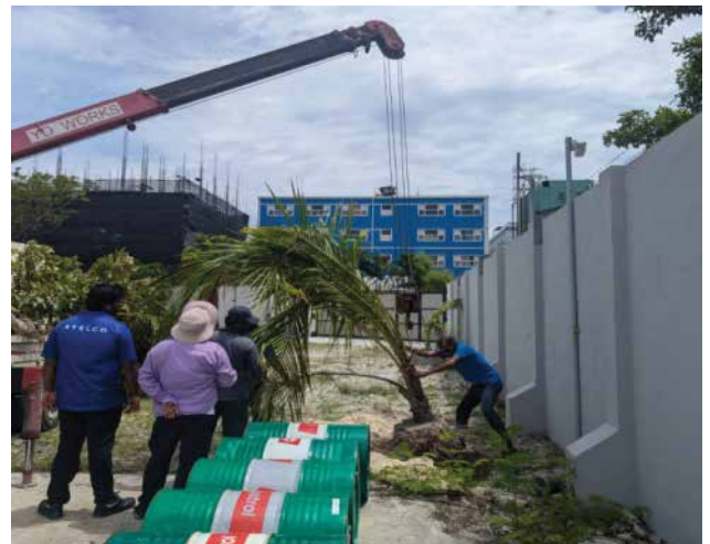
Figure 15 - Tree replantation during the land cleaning process, HulhuMale' Fifth Power Project
